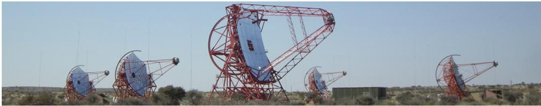
**Figure 1.3.:** The five telescopes of the H.E.S.S. instrument. The smaller CT1-CT4 are arranged along a square of 120m sidelength with CT5 in the centre.
