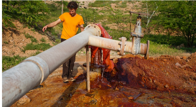
Figure A.11: Precipitated iron oxide on the ground at well Abu Zeeghan No 4
