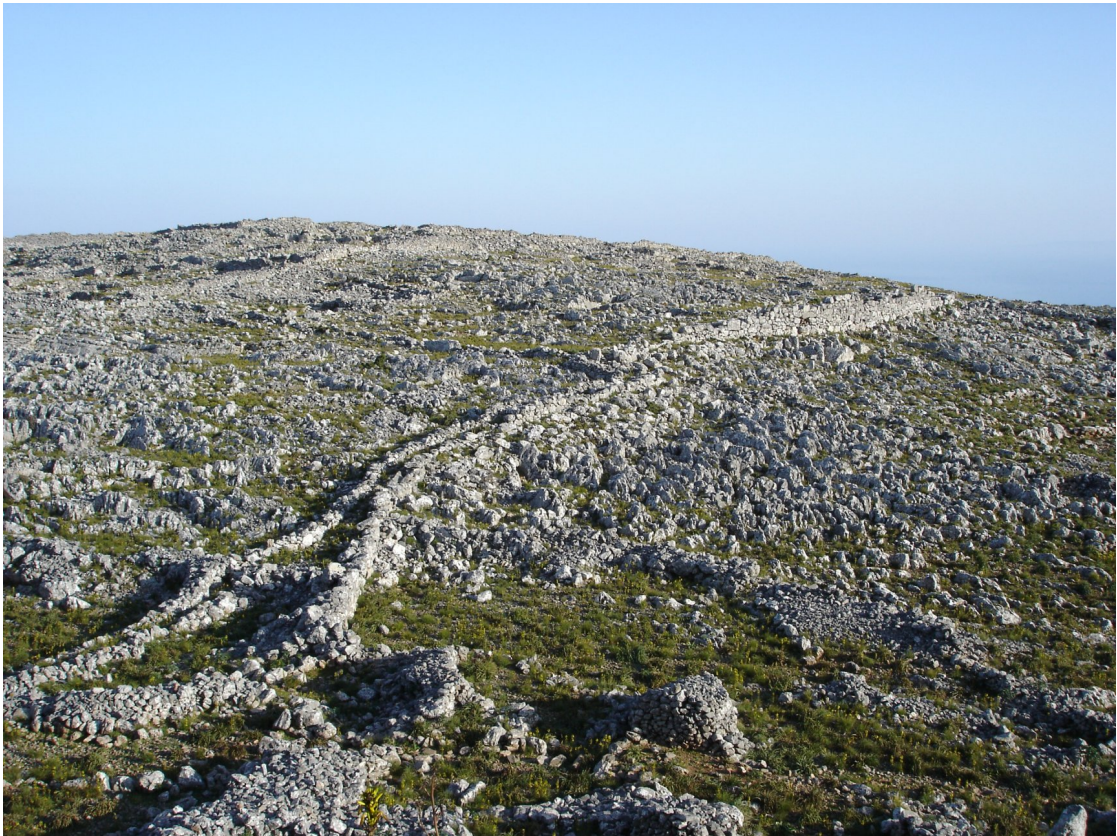
Figure 5.8: The western part of the city-walls of Anopolis, seen from south-west (April 2011)
