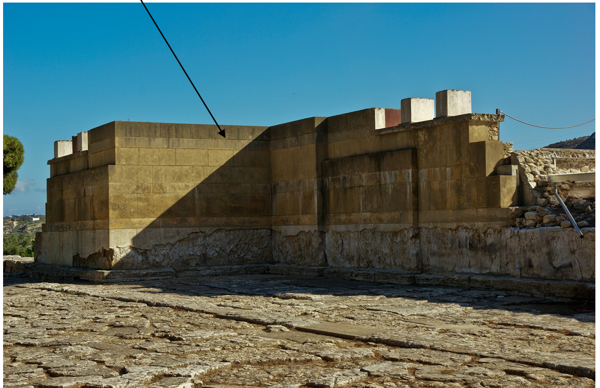
Figure 50 Detail of the West Facade at Knossos. Mark the Large Ashlar Blocks separated by Small Horizontal Bands.
