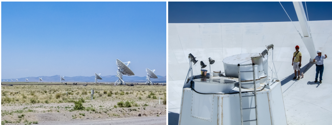
Figure 1.4: The left picture shows one arm of the VLA array including several antennas. The right picture illustrates the different receivers within one dish allowing a large coverage of different frequencies.
