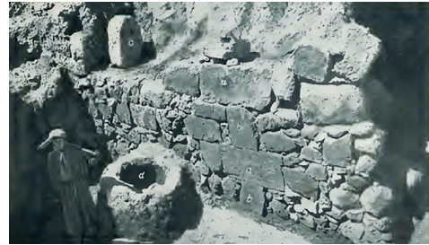
Fig. 28 Megiddo – Example of masonry with mixed headers and stretchers. SE room of the Palastwohnung, view from the NW (TM I A, Abb. 135)
