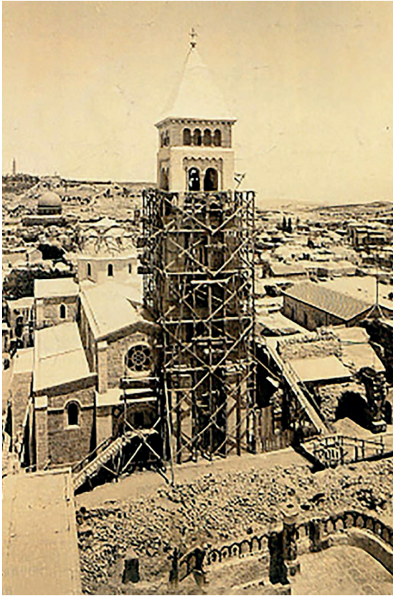
Fig. 1 Church of the Redeemer under Construction, Jerusalem 1896 (Carmel Eisler 1999)
