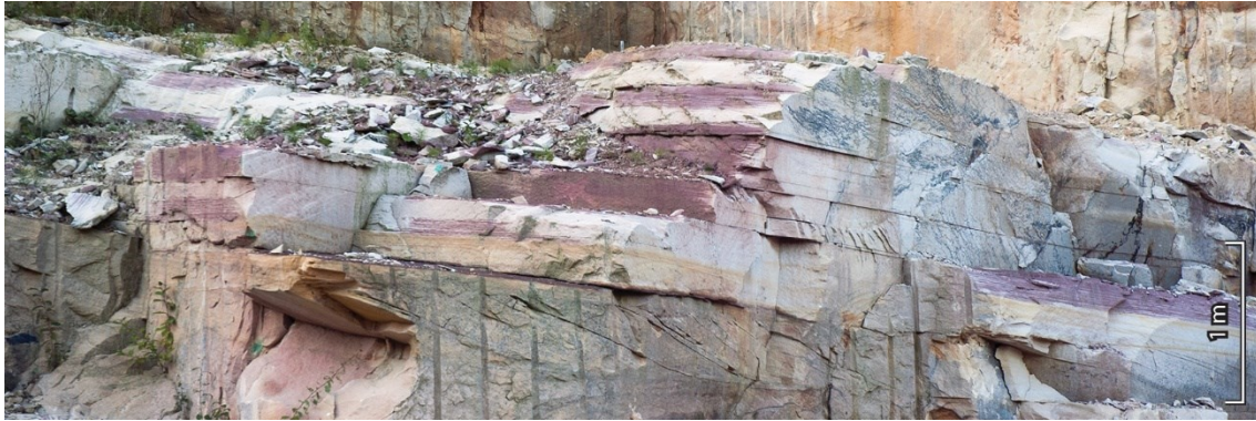
Figure 23: Yellow and white colors caused by bleaching within red sandstones, primarily along bedding planes and around fractures.
