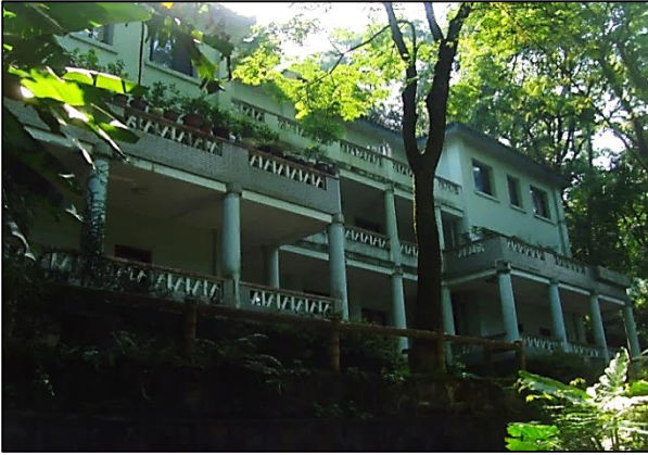
Figure 3.15. Façade of the Bolin Building. On the top floor the laundry is laid out to dry in the sun (Bonato, 2015)
