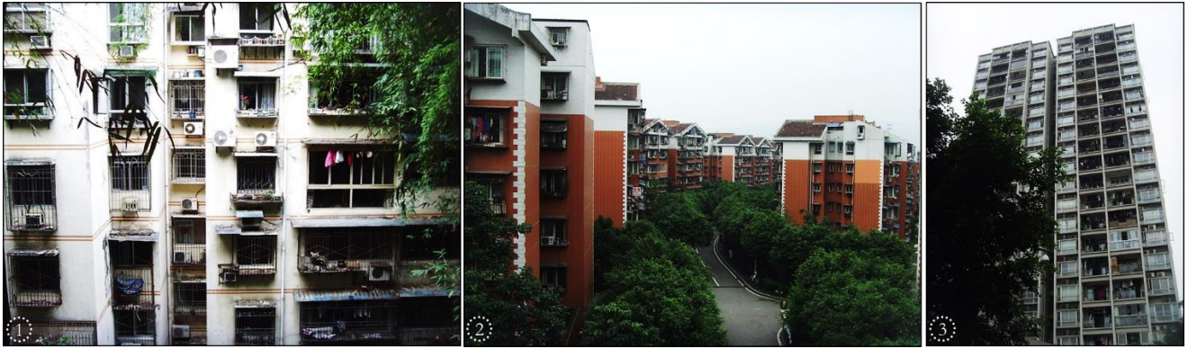
Figure 5.8. Affordable housing 1990s-2000s. 1) Housing model in Beibei Old Town; 2-3) Kangzhuang, Dazhulin Fanshequ “Big Bamboo Forest Model Community” in Yubei District, established in 2008 (Bonato, 2015)
