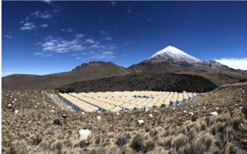
Fig. 3.1.: The HAWC Observatory in the National Park Pico de Orizaba in the Sierra Negra of Puebla, Mexico. The array is configured in a hexagonal shape, with avenues that allow access to each unit for maintenance purposes. The Pico de Orizaba seen in the picture is the tallest mountain in Mexico and the tallest volcano of North America. Image credit B. Dingus.
