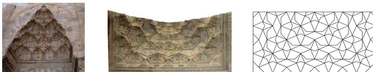
Figure 2.3. Portal to the enclosure at Sultan Han near Aksaray (Turkey). On the left: view from the front. In the middle: View from underneath. On the right: plane projection.
