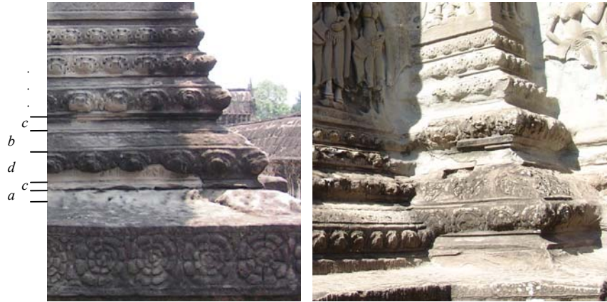
Figure 3.2.1 A special wall base structure: left, of the southern library of Angkor Wat's, and right, of Angkor Wat gopuram. Extraordinary location of b between d - and c -module in the sequence S_{LPE} = (a, c, d, b, c, d, c, d, c, d, c, a) .
