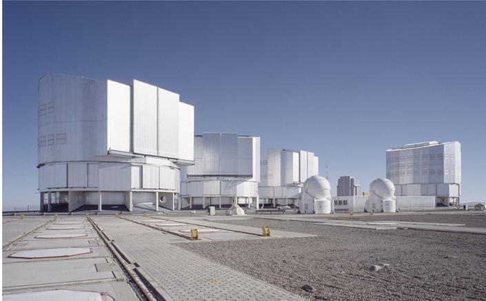
**Figure 2.13:** The VLT on Cerro Paranal. The picture shows the four UTs, two of the ATs, the interferometric laboratory (the flat building), the AT rail tracks and, in the background, the enclosure for the new survey telescope VST. The picture is taken from the ESO press release 06/05 (14<sup>th</sup> March, 2005) and has been slightly cropped to better fit the page. (<http://www.eso.org/public/outreach/press-rel/pr-2005/pr-06-05.html>)
